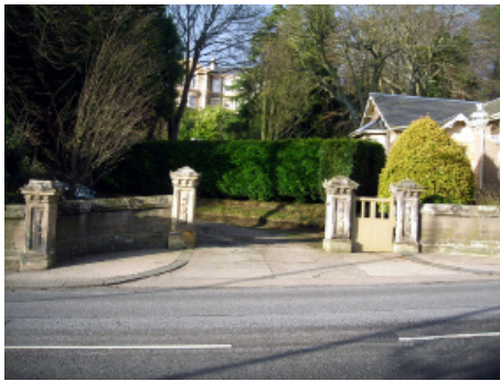
Decorative stone wall and gate piers
