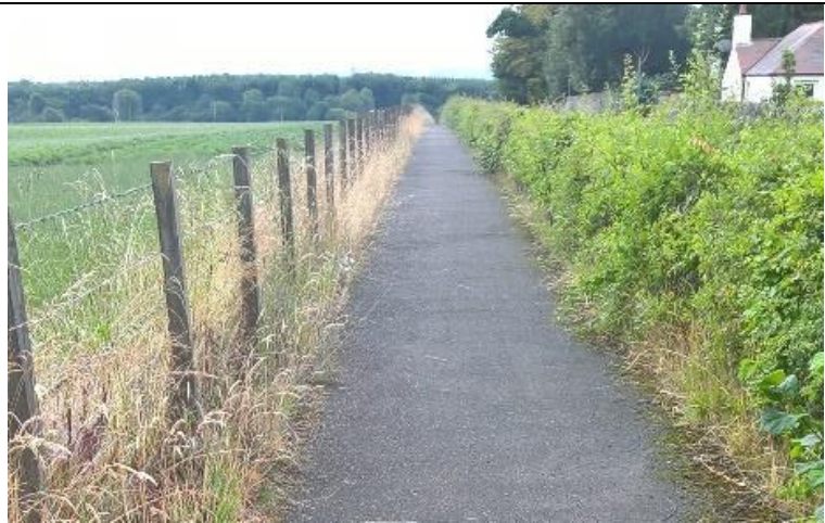
The constructed path alongside Dykes of Gray Rd
