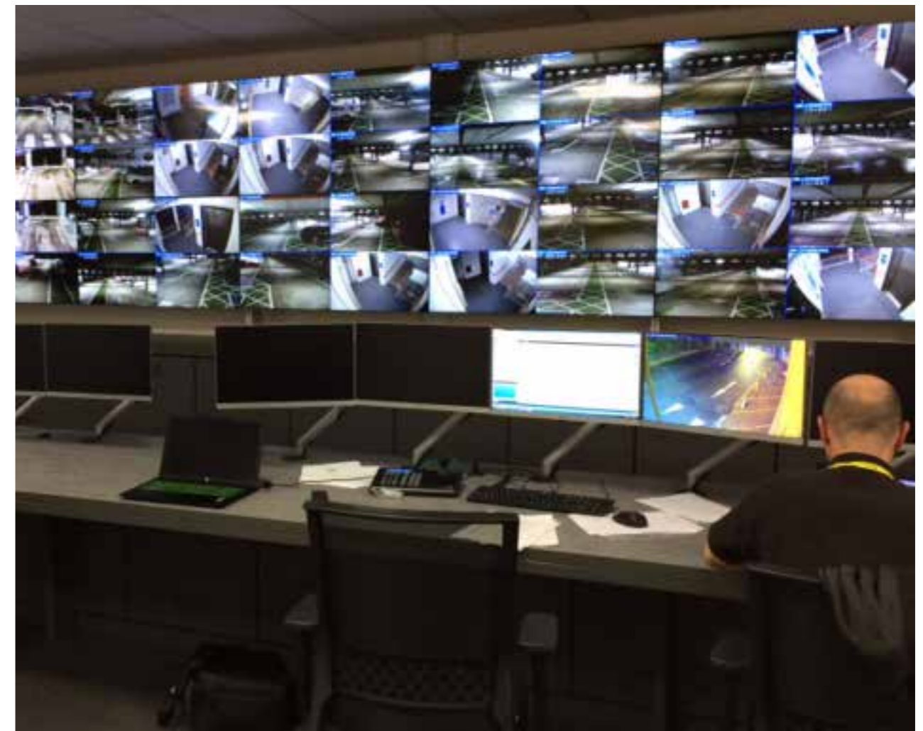
The Safety and Alarm Response Centre (SARC) became operational in April 2019. Housed within the West office in Lochee, the Centre can monitor up to 1200 cameras across the city, as well as several hundred alarm signals. The facility can also support the work of the Anti Social Behaviour Team and Community Safety Wardens and look forward to the expansion of the services provided by the team.
