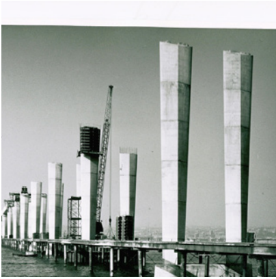
Tay Road Bridge Construction
