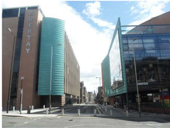
Above - View East along Bell Street
