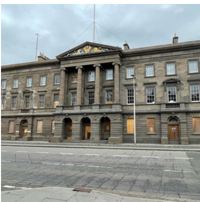
Former Customs House & Harbour Chambers Building
