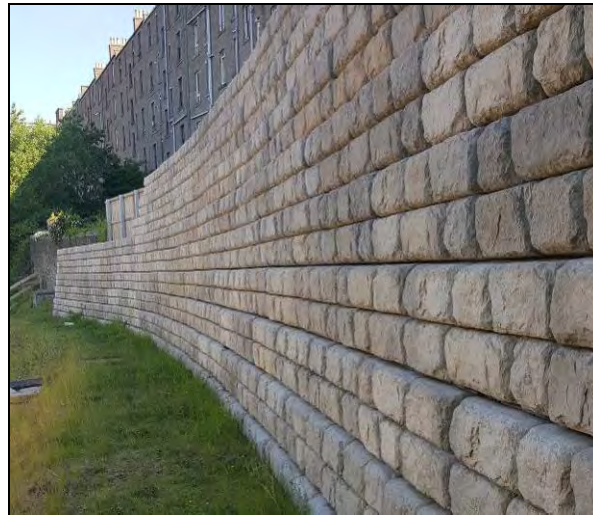
Photo 13 Example of Precast Concrete Retaining Wall
