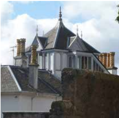
Roof detail and chimneys
