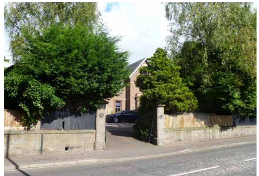
Boundary railings replaced with timber
