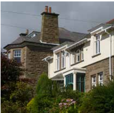
Roof detail and traditional windows
