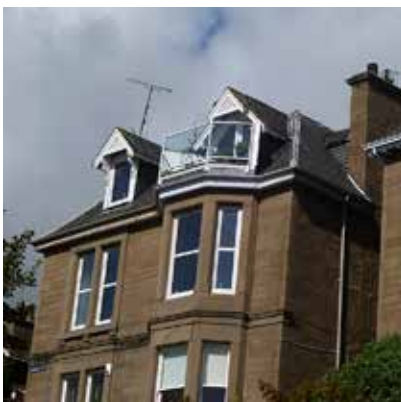
Traditional dormer windows and modern balcony
