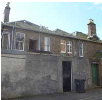
Sensitive wall repair
