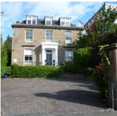
Traditional property within the Crescents Conservation Area
