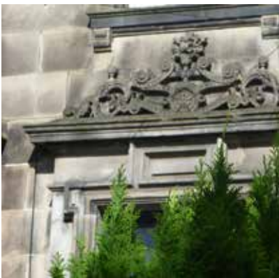
Architectural detailing adds to the character of the overall area
