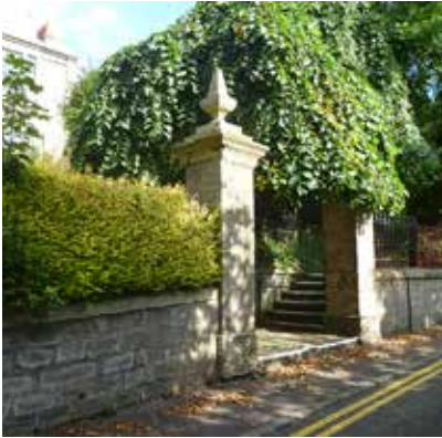
Hedges form part of boundary walls as well as the presence of mature trees
