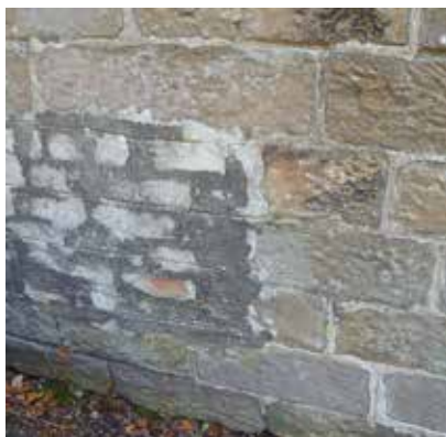
In insensitive wall repair
