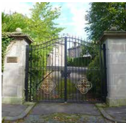
Traditional gate piers and gates
