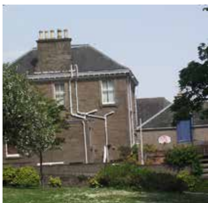
Back of house on Dalkeith Road as seen from the park
