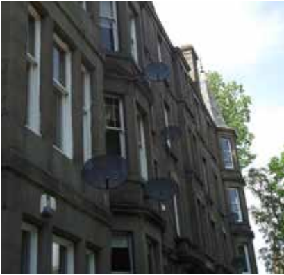
Clutter of satellite dishes on Baxter Park Terrace
