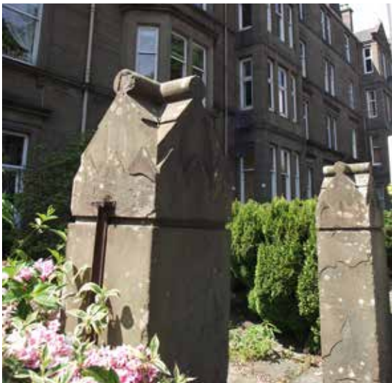
Gatepiers and boundary walls on Baxter Park Terrace
