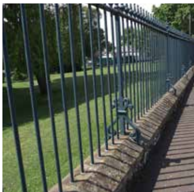
Section of original railings on Wortley Place
