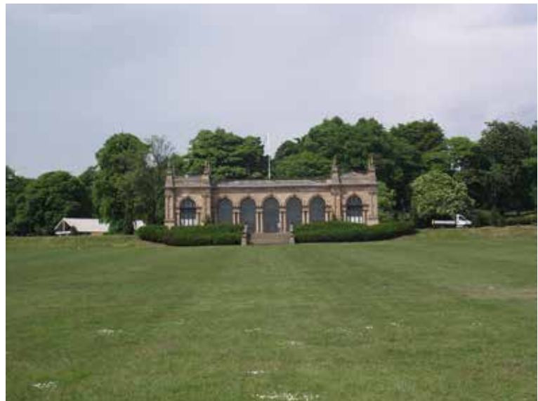
View of the pavilion from the parade ground
