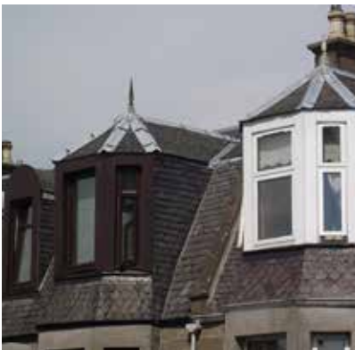
Slate roofs with modern windows on Wortley Place
