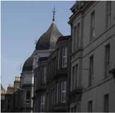
Slate roofs on Arbroath Road
