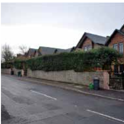
Duntrune Terrace New Build
