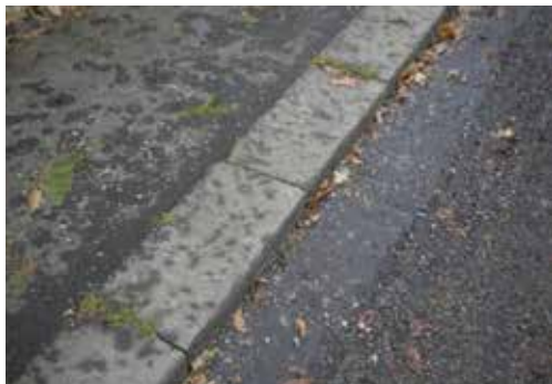
Wide stone kerb with stone drainage channel
