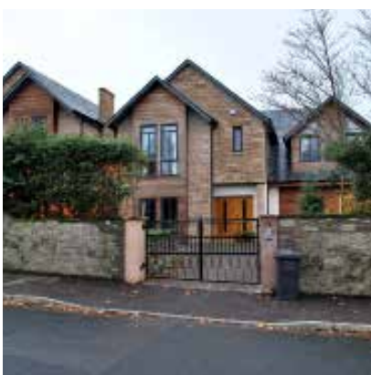
Duntrune Terrace New Build
