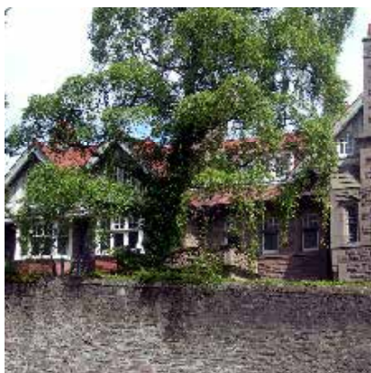
Aystree seen behind high boundary wall
