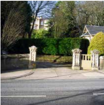
Decorative stone wall and gate piers
