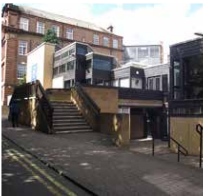
Bonar Hall entrance from Park Place
