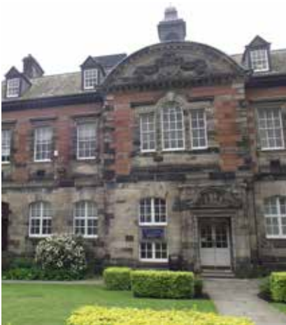
Carnegie Building facing Geddes Court
