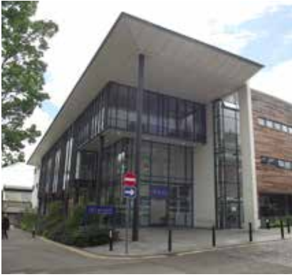
Main Library Modern Frontage
