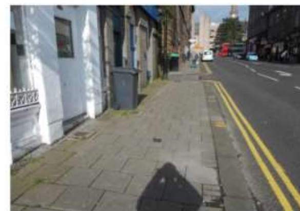
Precast concrete slabs on St Andrew's Street
