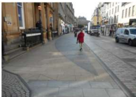
Older sections of Silver Aberdeen Townscape amongst the more recent Grey Chinese Granite.
