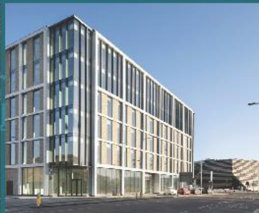
The Central Waterfront's new Earl Grey Building. Social Security Scotland will be the first tenants, with space for up to 600 employees.
