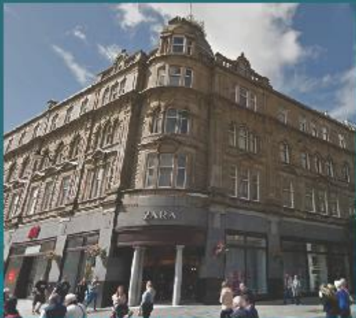
Upper floor residential opportunities on the corner of Commercial Street and the High Street.
