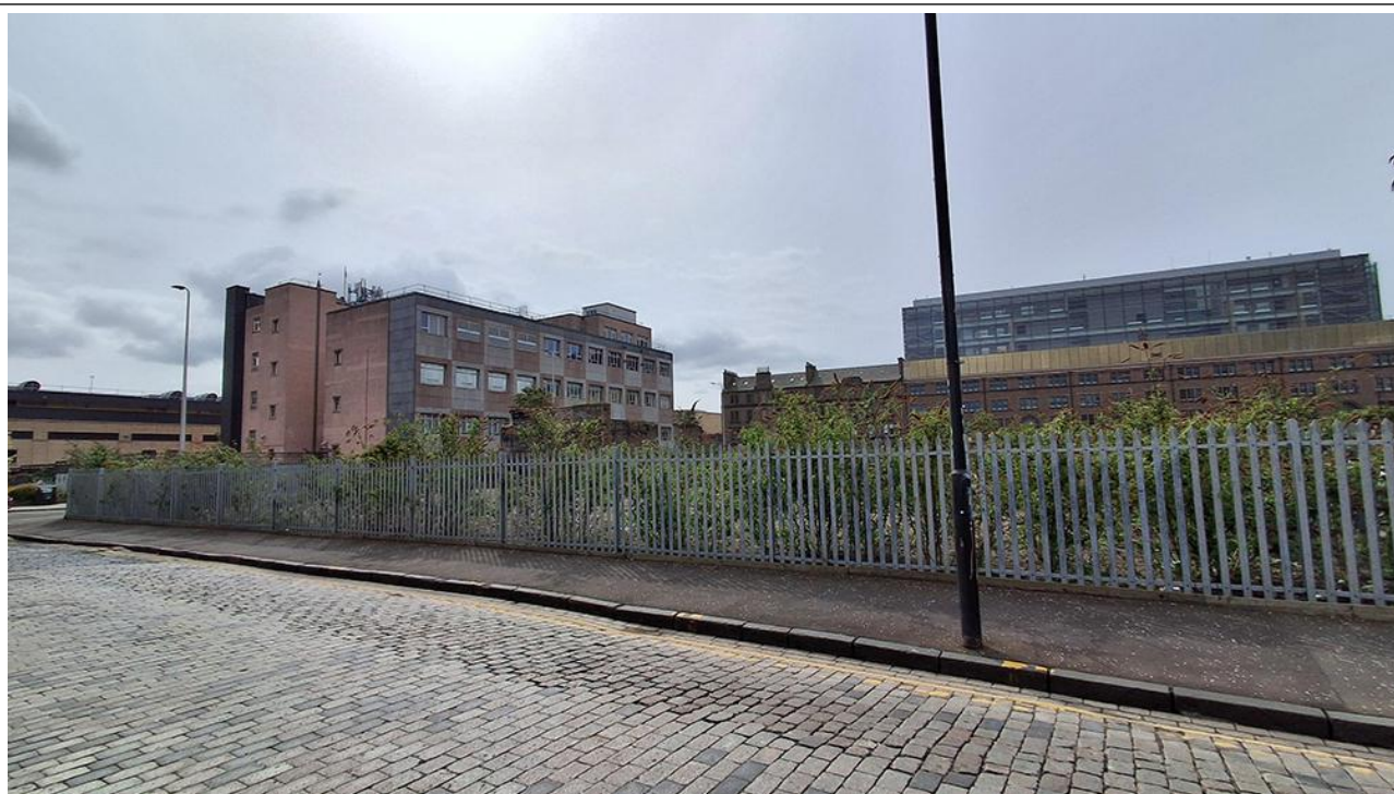
Figure 3: View of Site From Barrack Street
