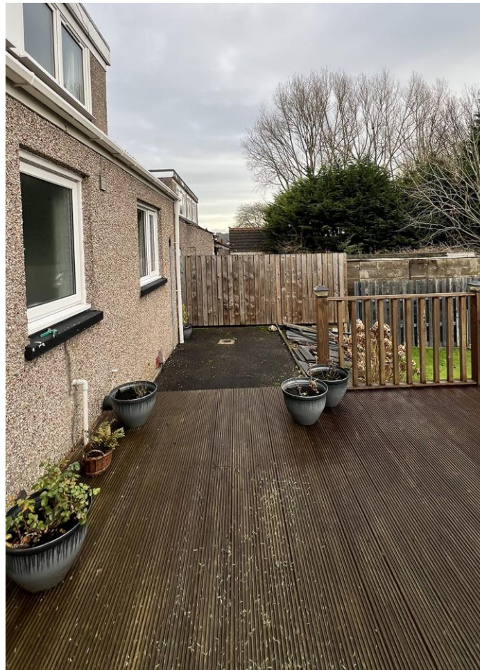
Figure 6 – Rear of House Facing East
