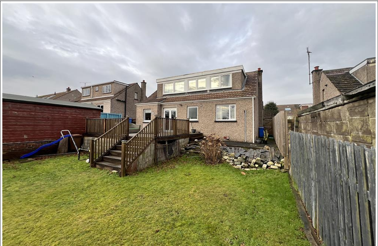
Figure 3 – Rear of House Facing North
