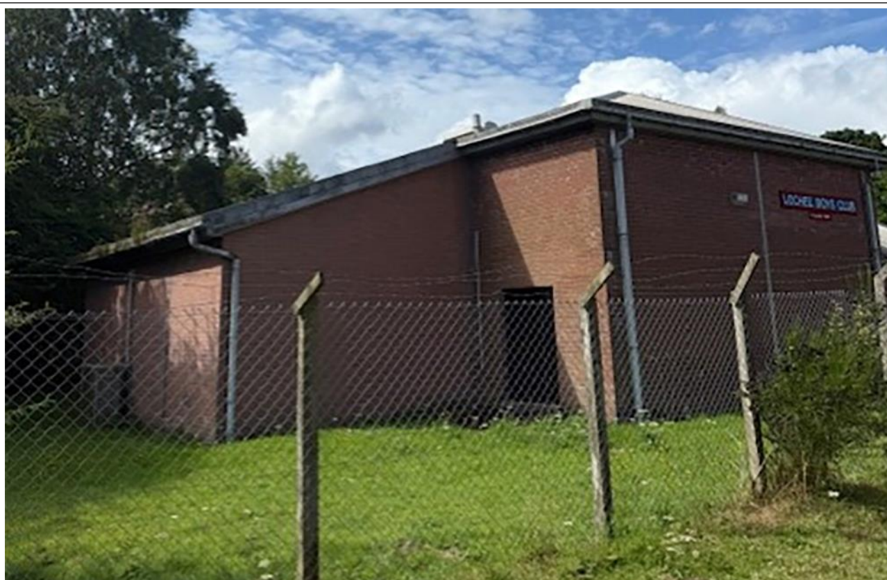
Figure 4 – Rear of Building and Boundary Fence
