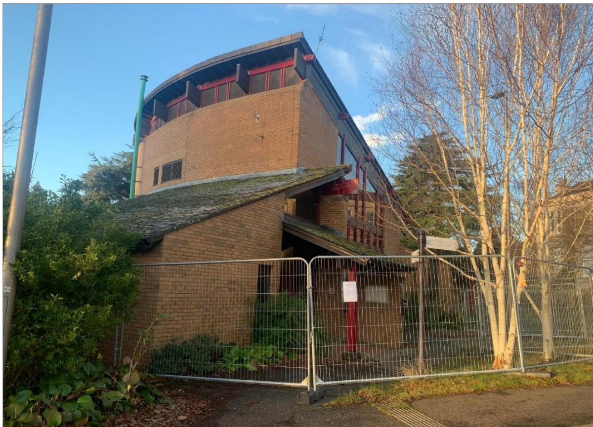
Figure 5 – View of Existing Building
