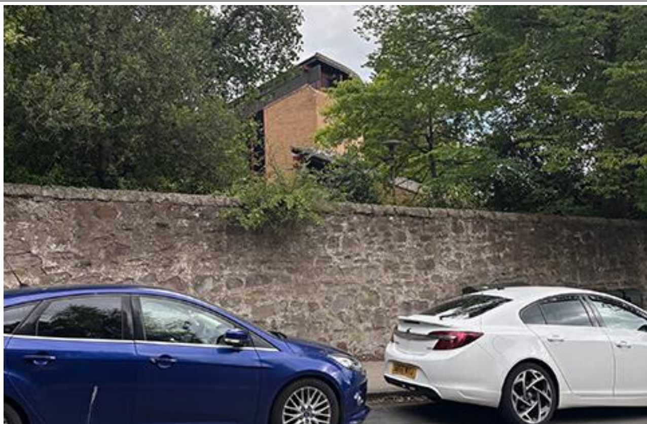
Figure 4 – View From West Park Road Looking East
