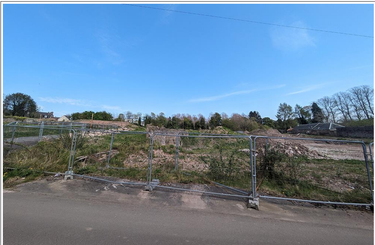
Figure 4 – Looking west across the site
