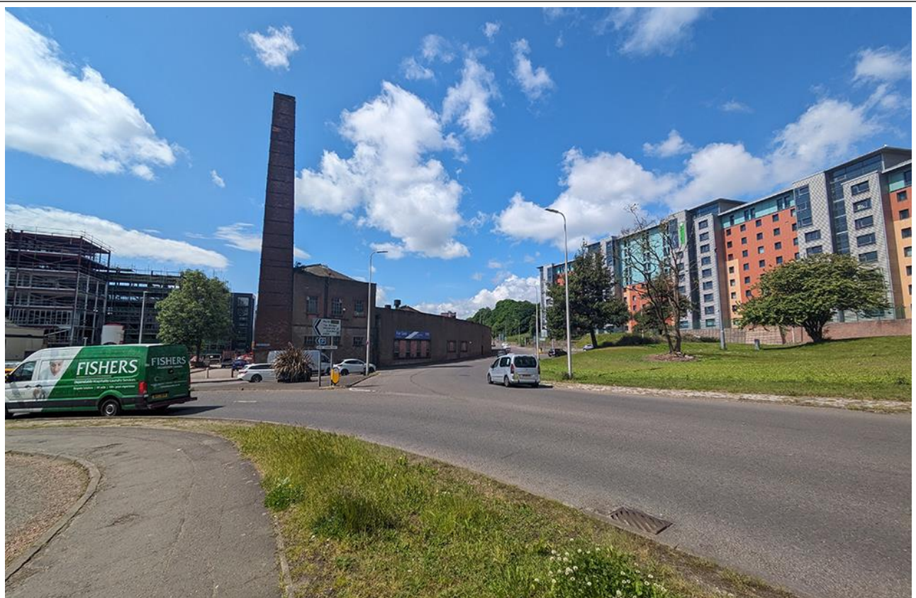
Figure 3 – View Looking Across West Marketgait to Locarno Works
