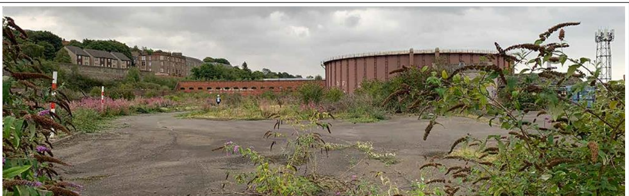
Figure 12 – Image From South of Site Looking Across to Gas Holder
