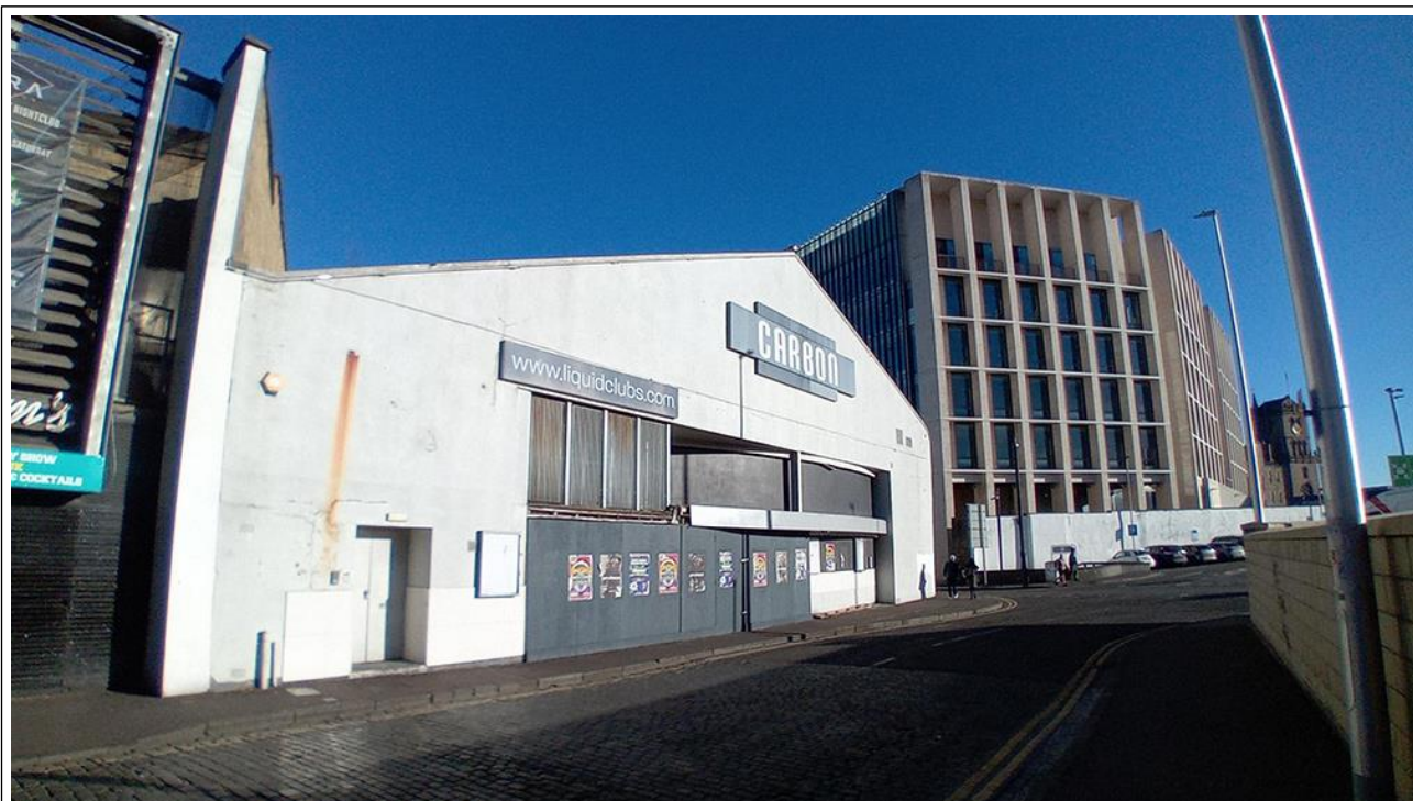
Figure 3: View of Site From Johnston Street
