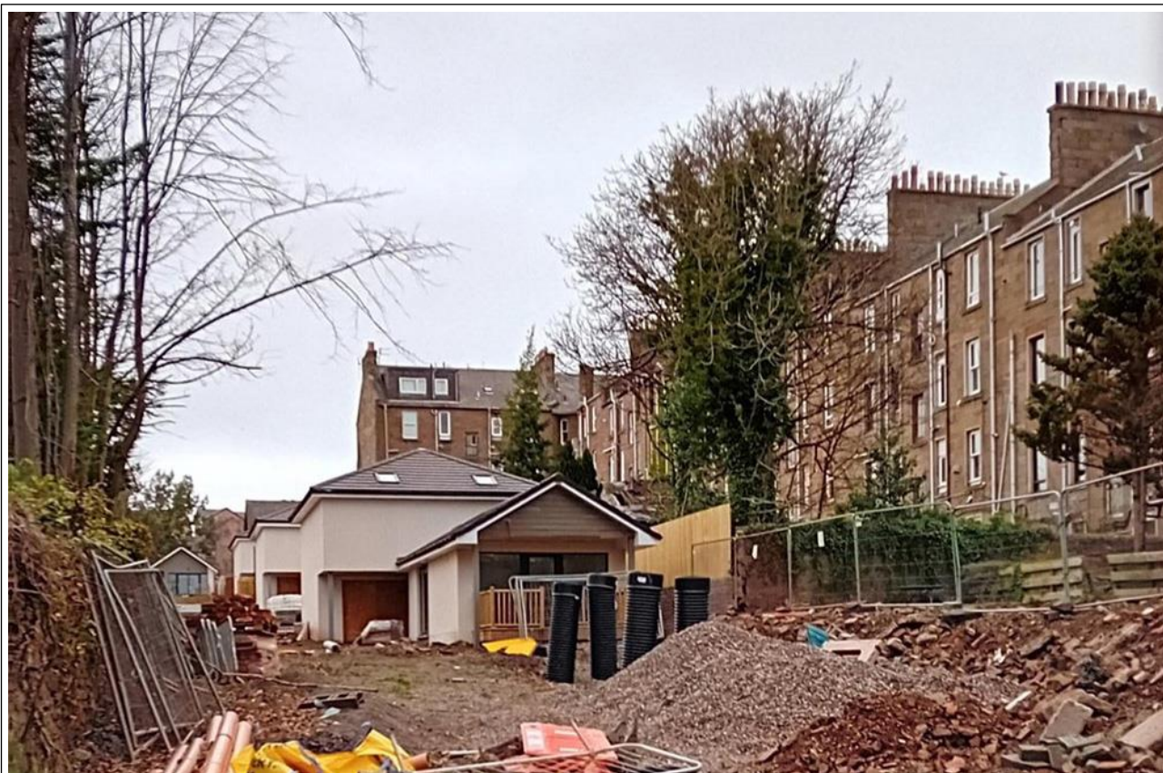
Figure 6: View of Site From Magdalen Yard Road
