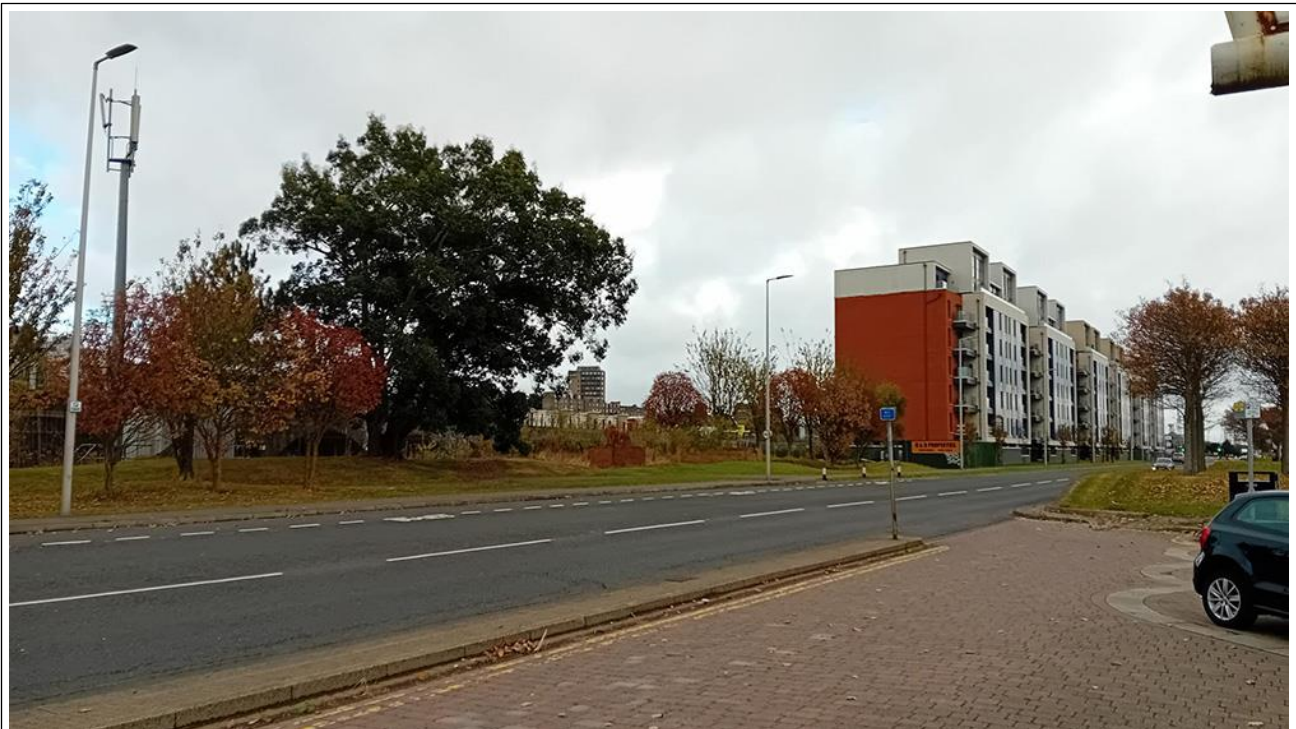
Figure 6: View of Site From Riverside Drive
