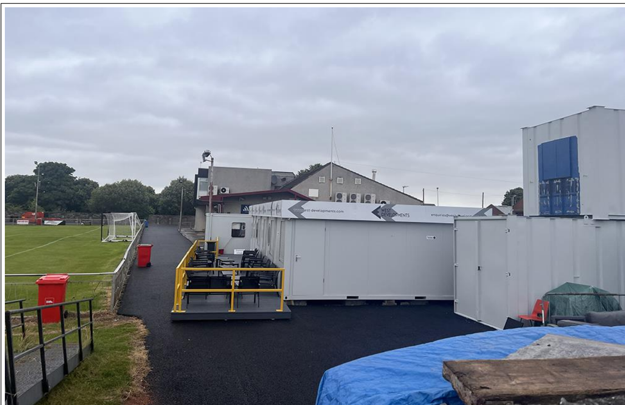
Figure 3 – South Elevation of Modular Buildings
