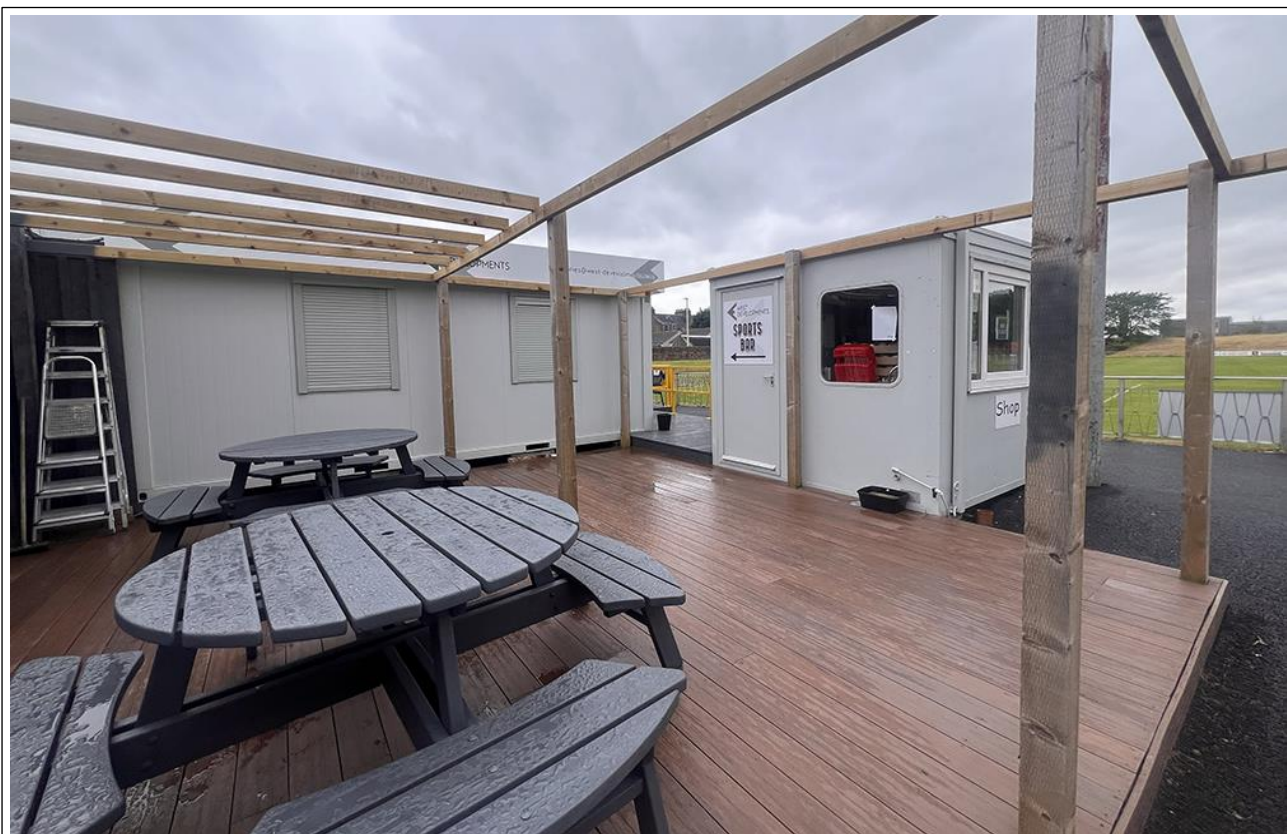
Figure 4 – Decking on North Side of Modular Buildings
