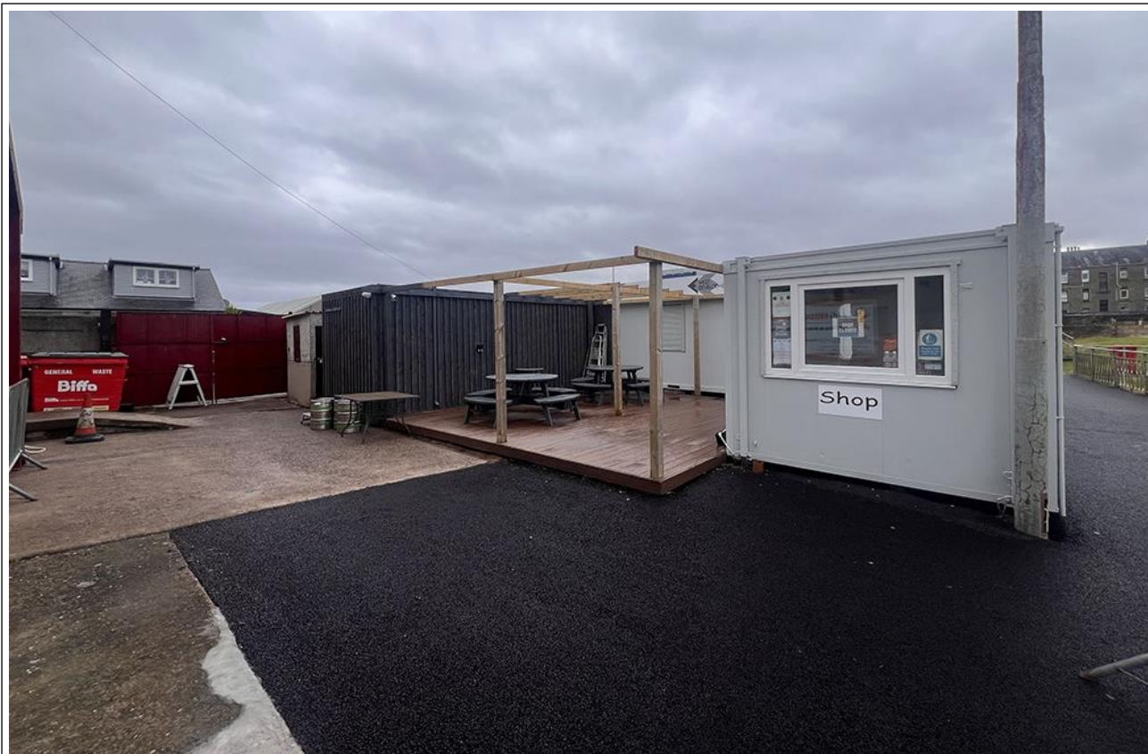
Figure 5 – North Side of Modular Buildings
