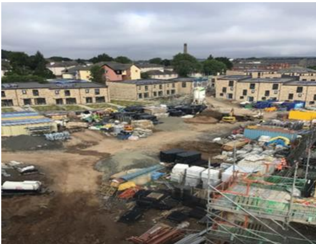
Ongoing development at Derby Street (Hillcrest HA).
