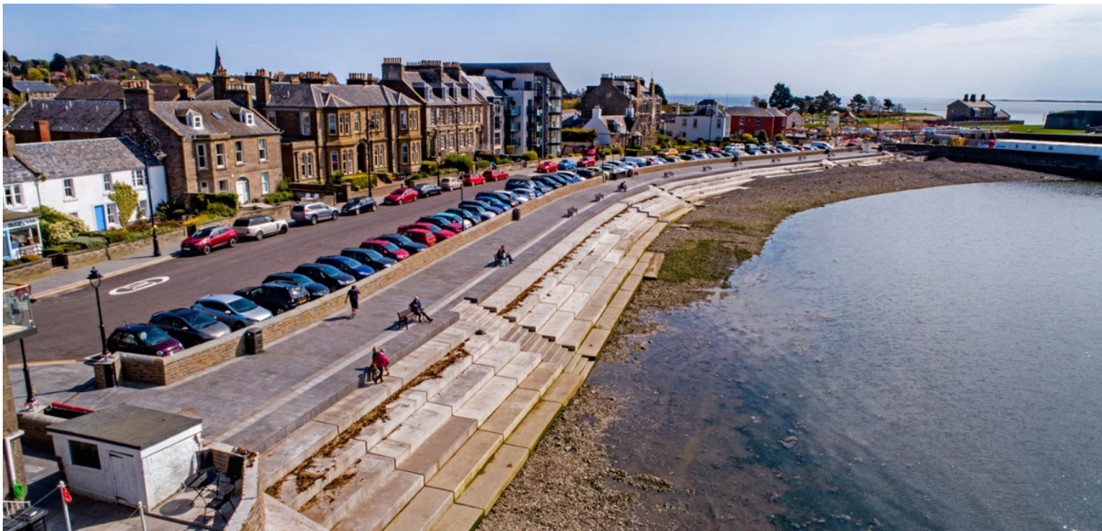
Image: Broughty Ferry Flood Protection Scheme and Active Travel Scheme
