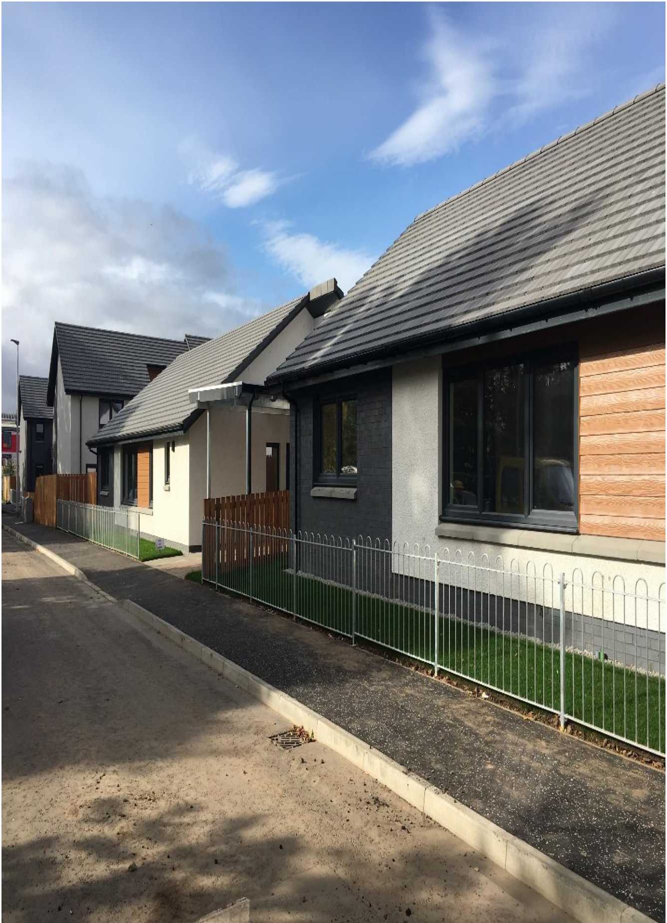
New Build Wheelchair Housing Alexander Street
