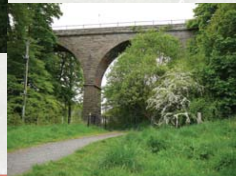
The Seven Arches Viaduct
