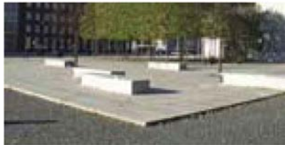
Raised kerb defines trafficable zone
