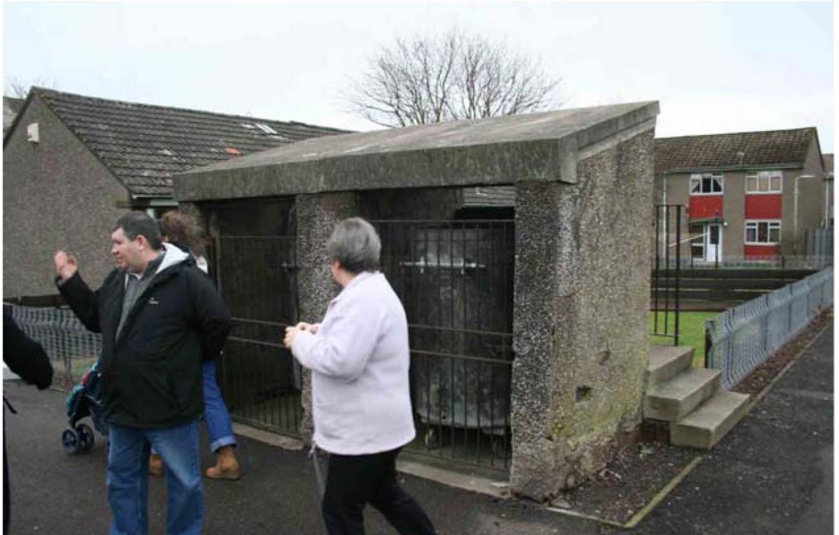
Existing communal bin storage in Mill O' Mains
