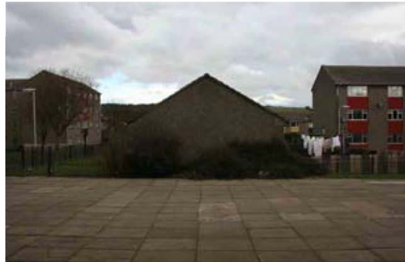
Hard landscaped areas poorly overlooked
