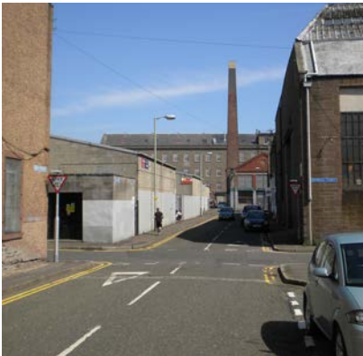
View along Miln Street
