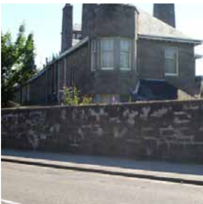
inappropriate repairs to boundary wall
