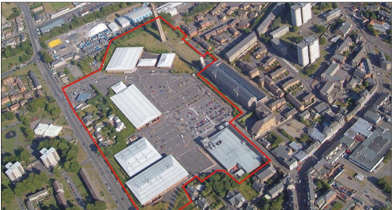
Figure 9 - Aerial Photograph of Stack Leisure Park
