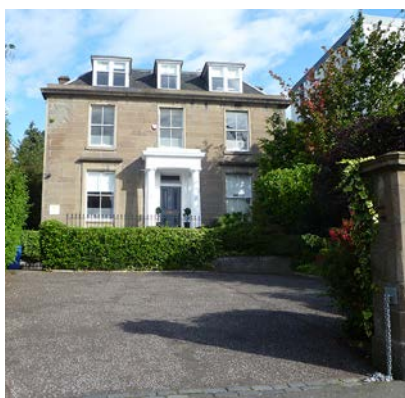
Traditional property within the Crescents Conservation Area
