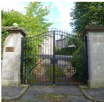
Traditional gate piers and gates
