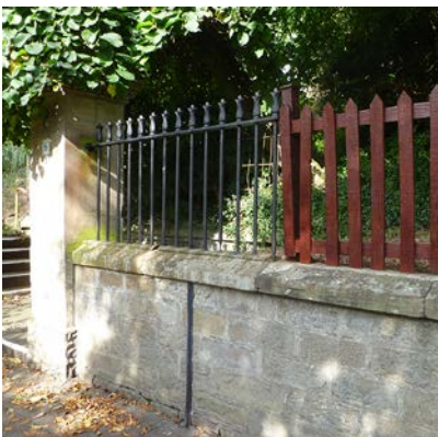
Some iron work has been replaced with timber fencing. This is taking away character from the area
