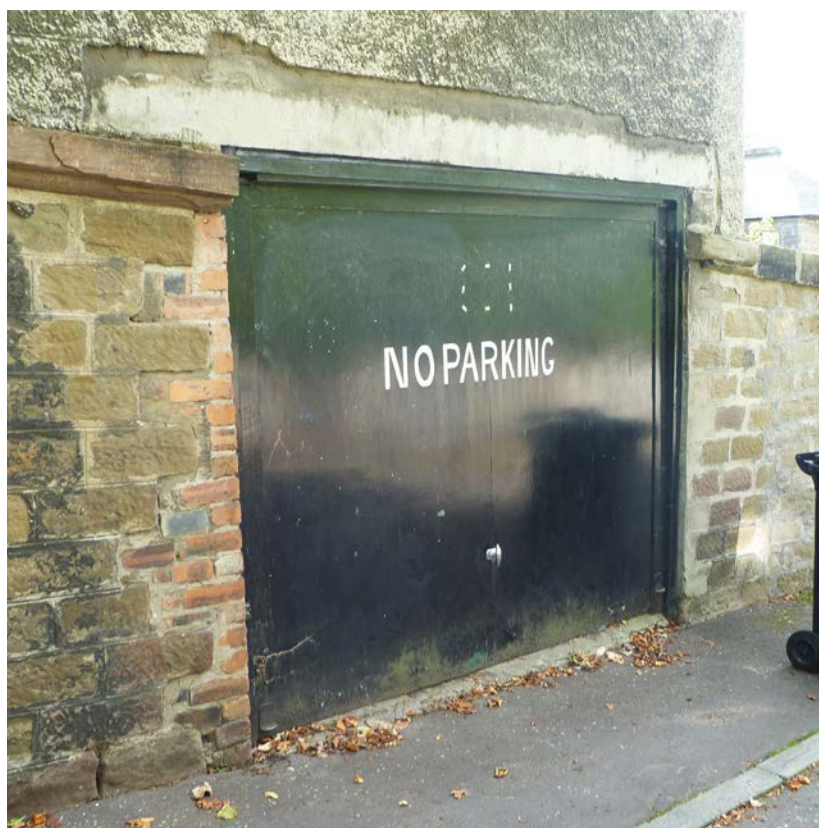
Partial loss of boundary walls for garages and parking causes detrimental effects on the area's character
