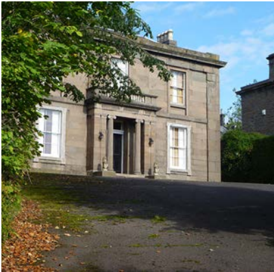
The majority of villas within the conservation area are listed by Historic Scotland
