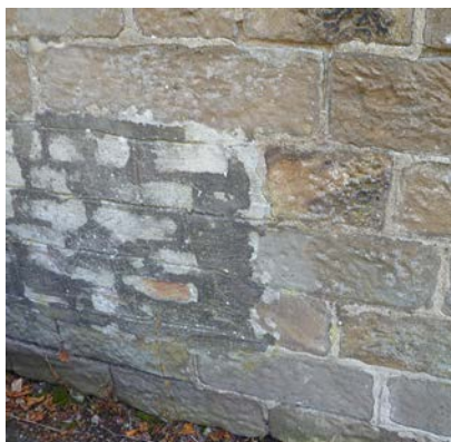
In insensitive wall repair
