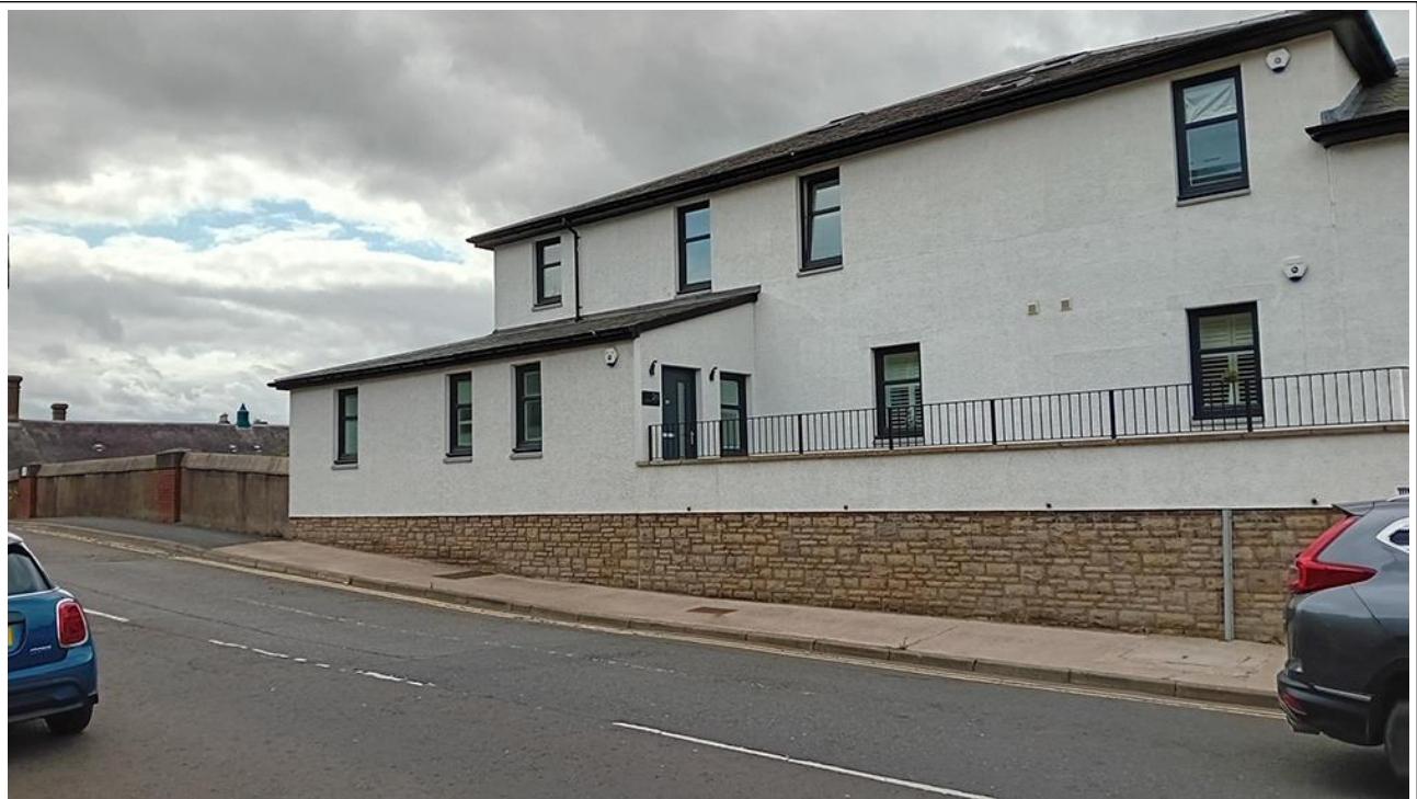
Figure 3 – View of Site From West Queen Street
