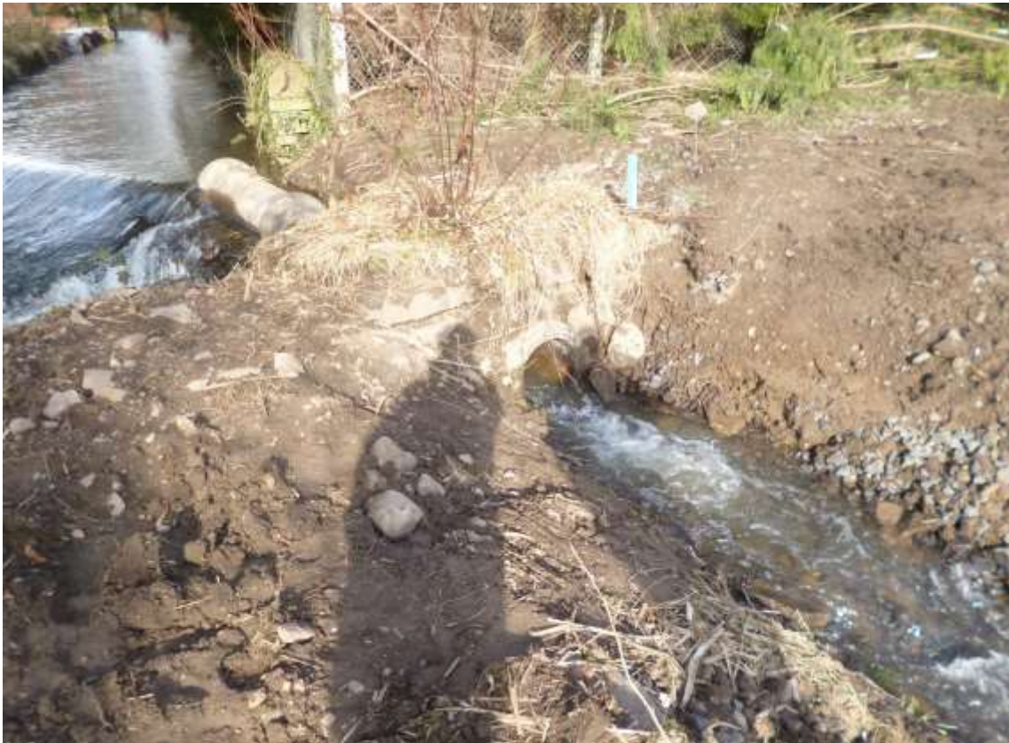
Figure 3 – Site Photo showing Weir and Inlet Pipe (March 2018)
