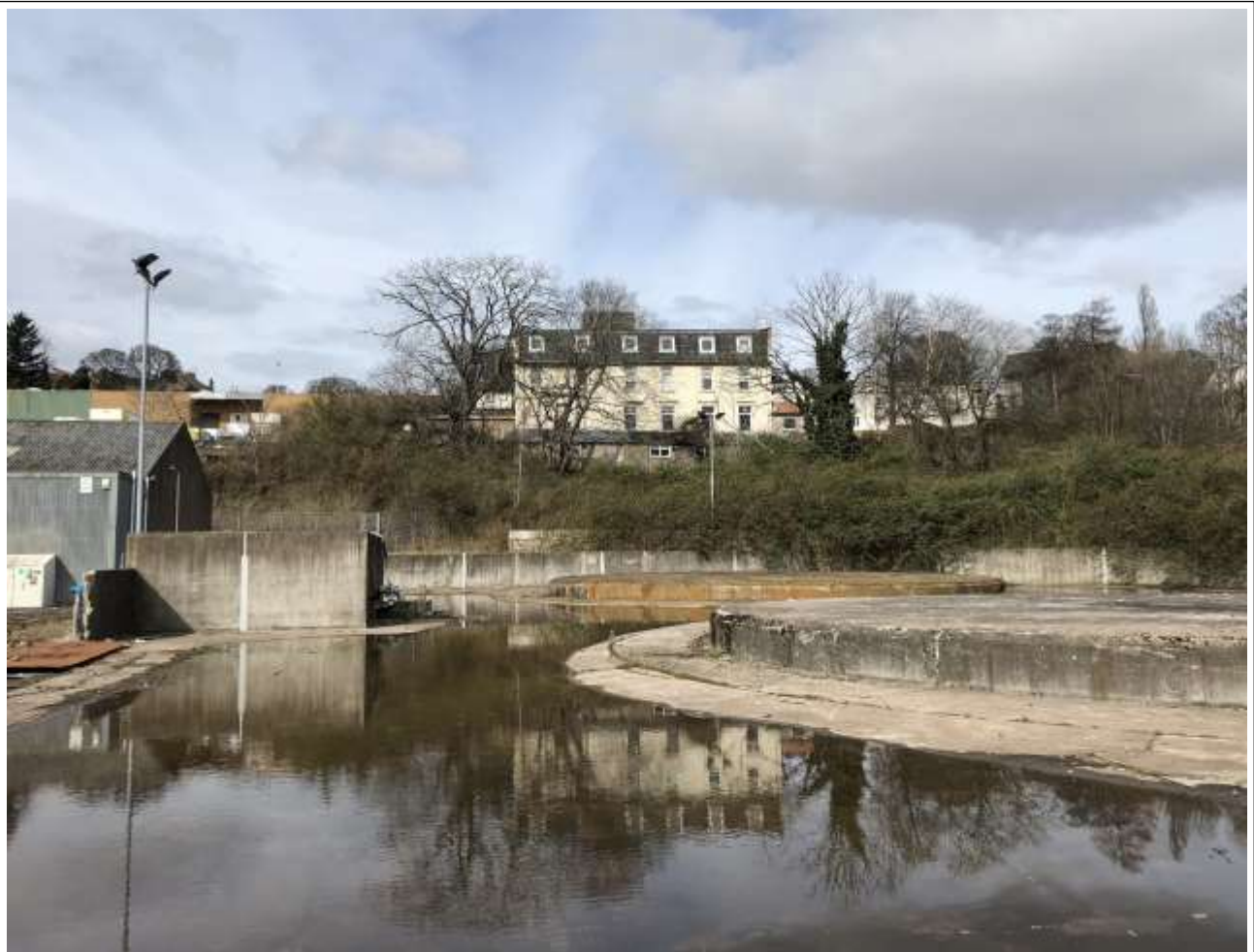
Figure 2 – Photo of Site
