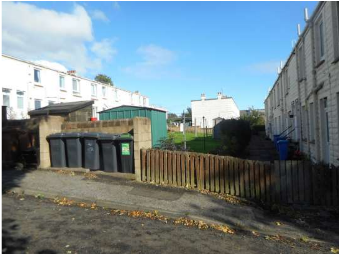
Figure 7 – Photo of Existing Houses on Ellengowan Drive (west)
