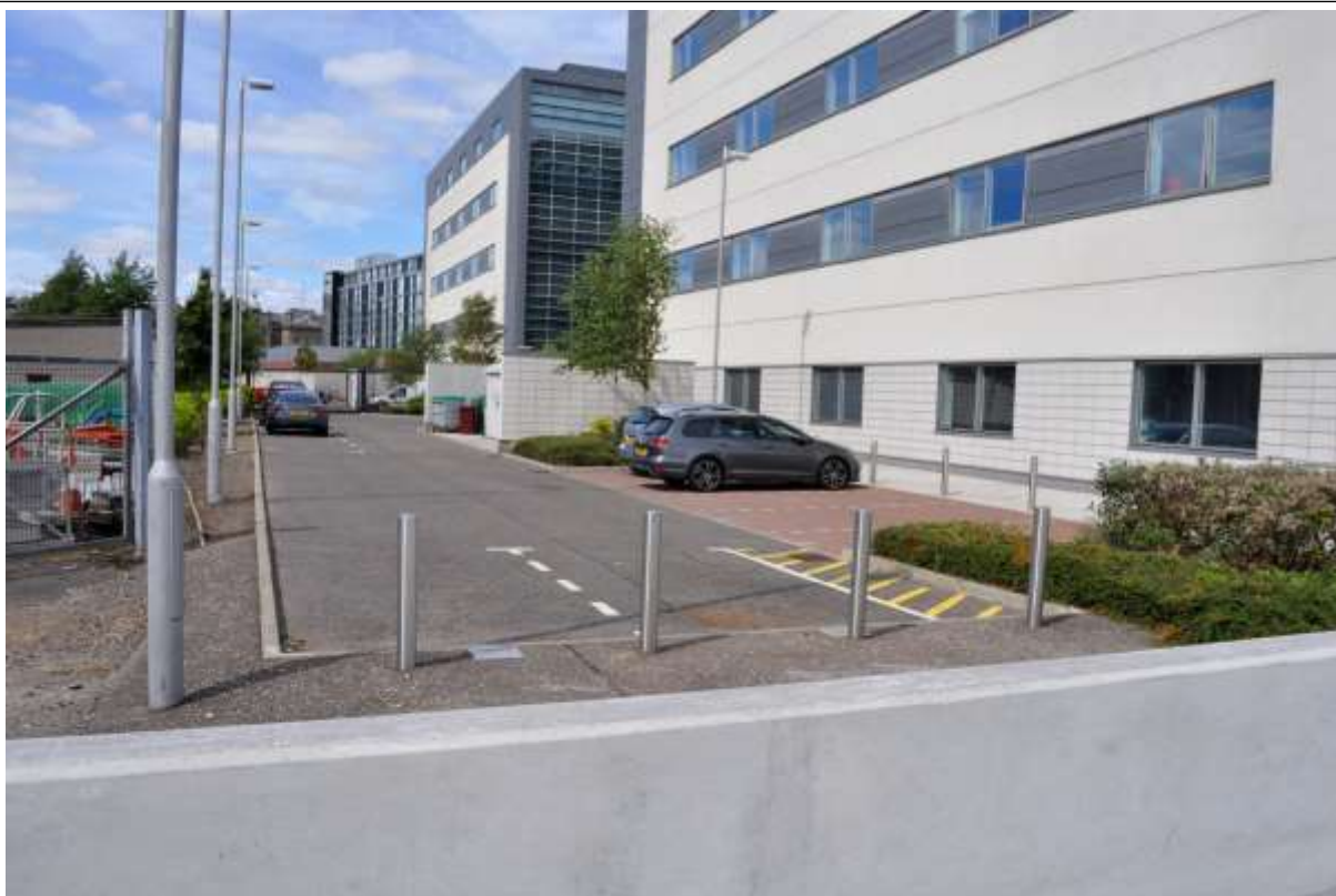
Figure 4 – Existing Landscaping to East of River Court (View North)
