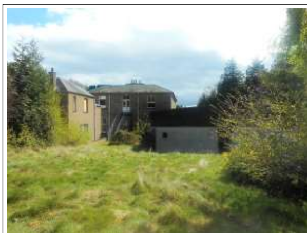
Figure 3 – Anton House – Rear Elevation
