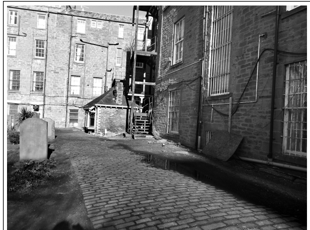
Figure 5 – Existing Rear Elevation
