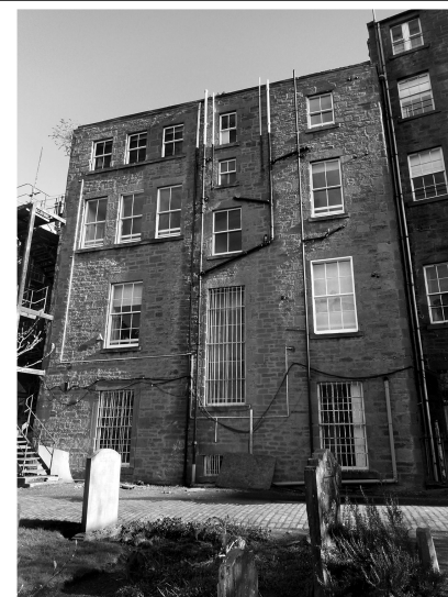
Figure 3 – Existing Rear Elevation
