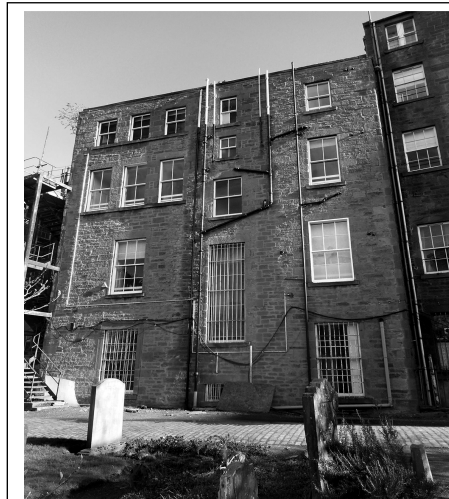
Figure 3 – Existing Rear Elevation
