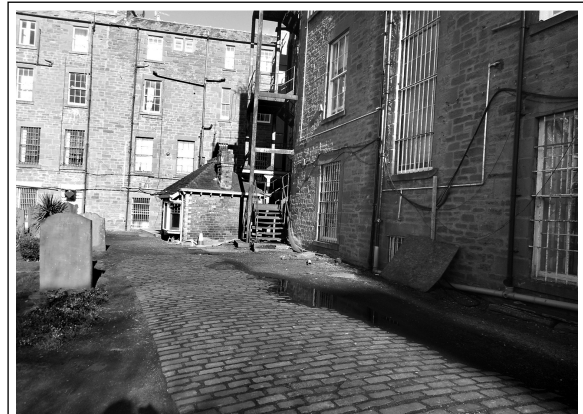
Figure 6 – Existing Rear Elevation
