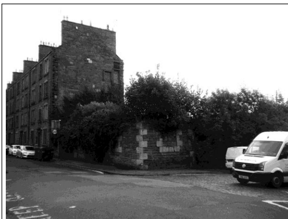
Figure 3 – Photo Looking East on Mollison Street
