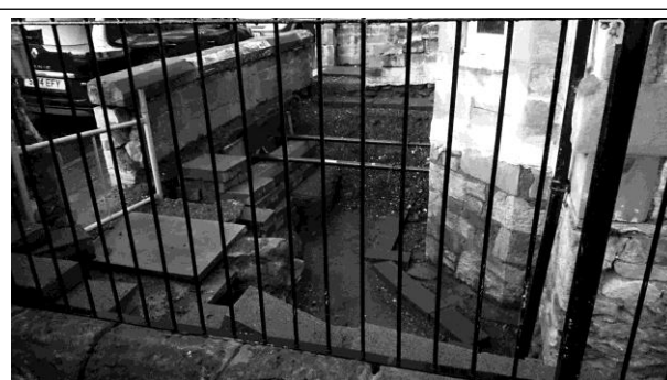
Figure 3 – Photograph of Excavated Front Garden, Including South and West Boundaries
