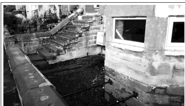
Figure 2 – Photograph of Excavated Front Garden
