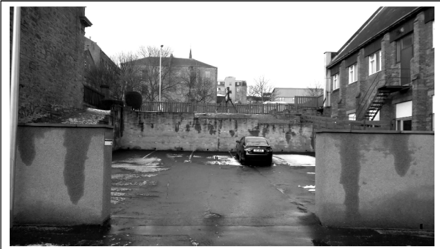
Figure 5 – Photo From The South
