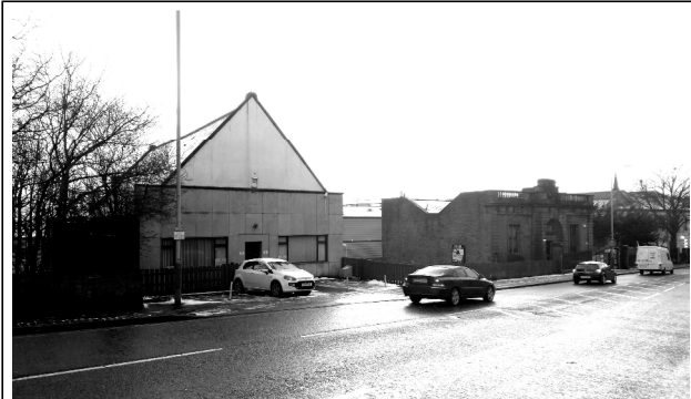
Figure 4 – Photo From the North
