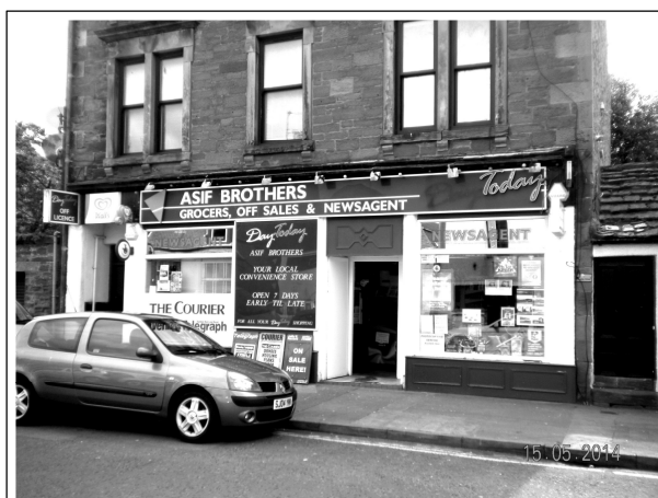
Figure 3 – Photo of Existing Shopfront
