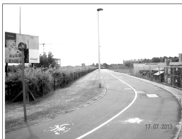
Figure 3 – Existing Cycle Footpath
