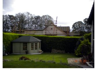
At present the original house is being redeveloped with a partially completed flat roof extension being erected on the eastern elevation of the house. Changes have also been made to the southern elevation with the existing/ enlarged window openings covered with timber boards. The original roof tiles have been stripped of the remaining pitched roof and the dormer extension.
