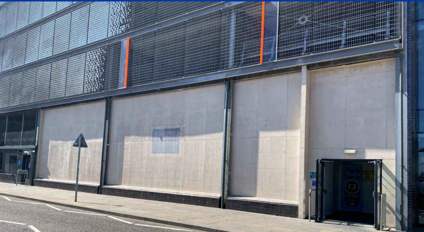
East elevation overlook Gallagher Retail Park
